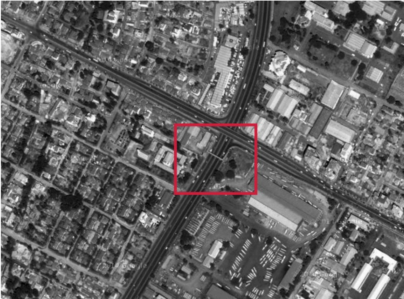
fig. 60: perimeter extension site 2
