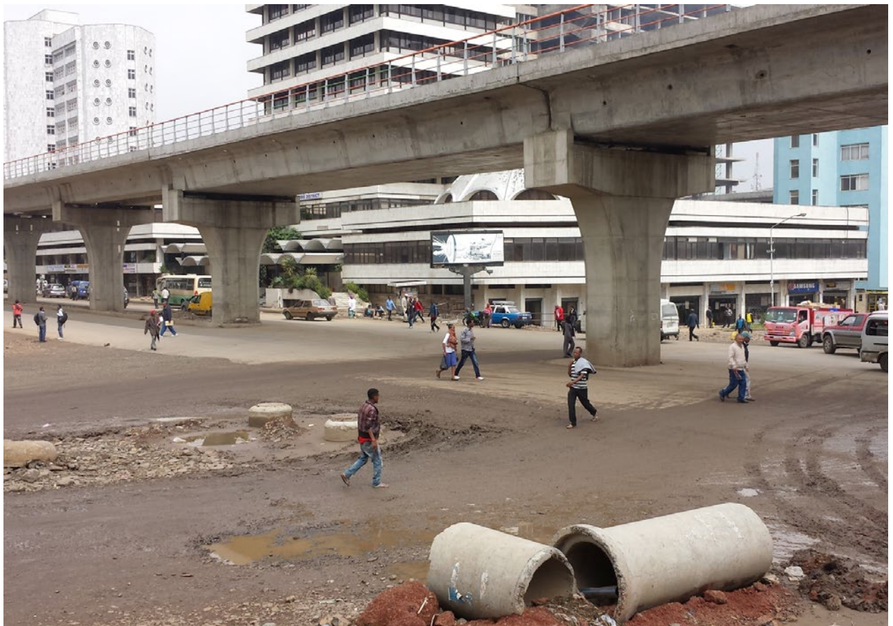
fig. 36: current pedestrian infrastrucutre at La Gare intersection
