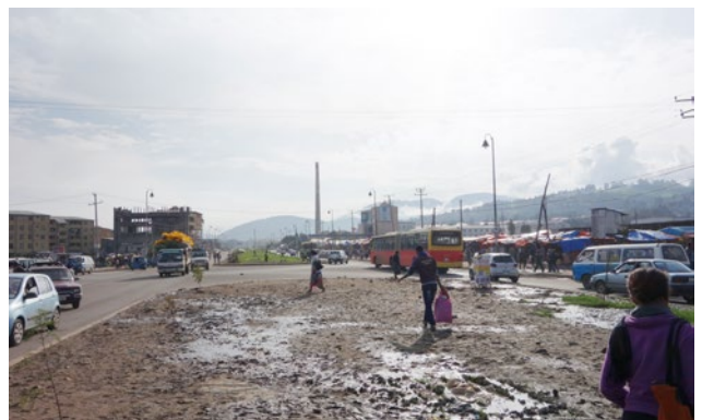
fig. 76: mud terrain on the intersection
